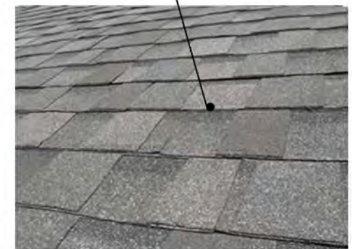
architectural shingle roof
