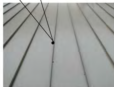
standing seam metal used as siding
